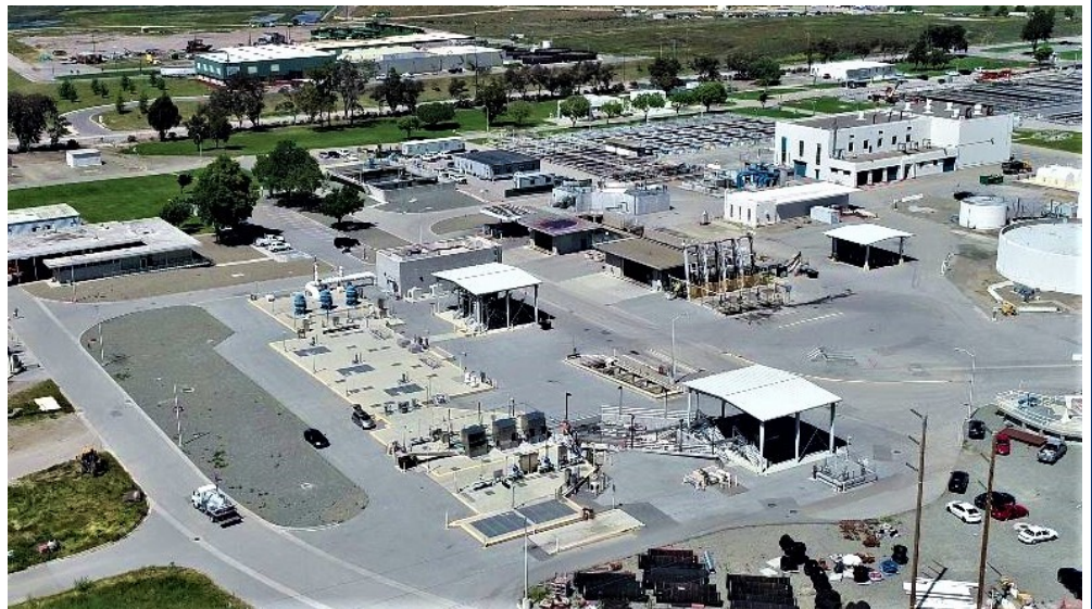
Headworks Critical Improvements
