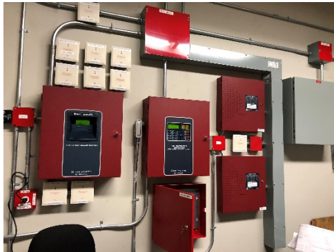
* PAC Fire Alarm System Replacement
