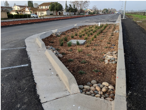
* Chynoweth Avenue Green Street Project
