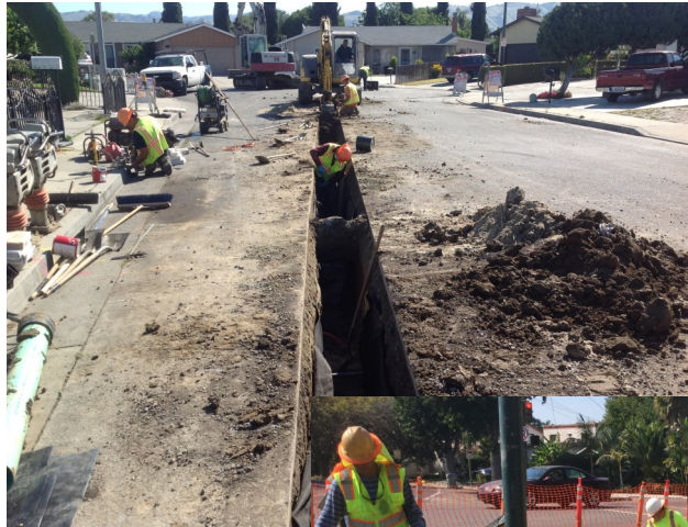
Tolbert Ct. Sanitary Sewer Cast Iron Replacement
