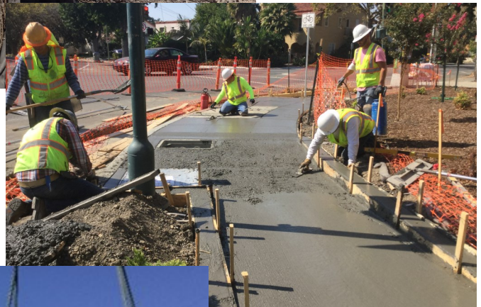
Park Avenue Multimodal Streetscape Improvements
