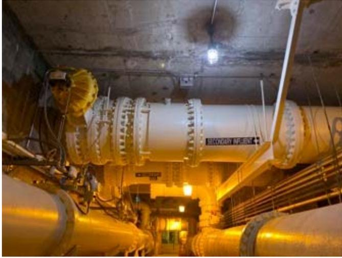
Figure 6: New Secondary Settled Sewage Influent Magnetic Flow Meter
