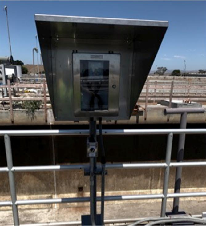
Figure 8: New Dissolved Oxygen Transmitter at the Secondary Aeration Basins
