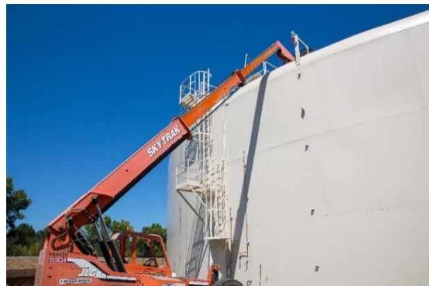
Detail Work on Trimble Reservoir
