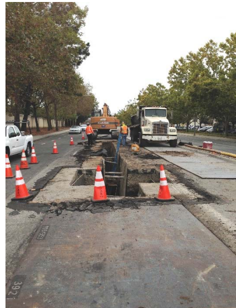
Coleman Road Sanitary Sewer Replacement
