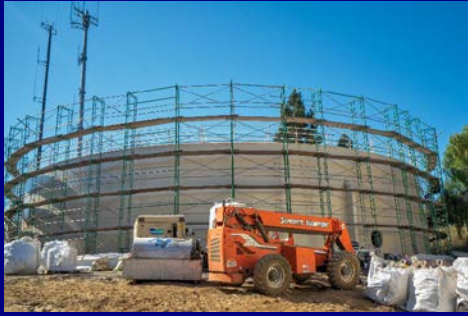
Cadwallader Tank Exterior
