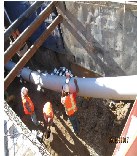
Williams Rd – Moorpark Ave Sanitary Sewer Improvement
