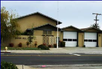
Major Repairs at Fire Stations 3, 9, and 30
