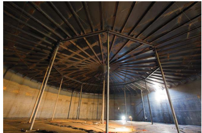
Interior of Cadwallader Reservoir
