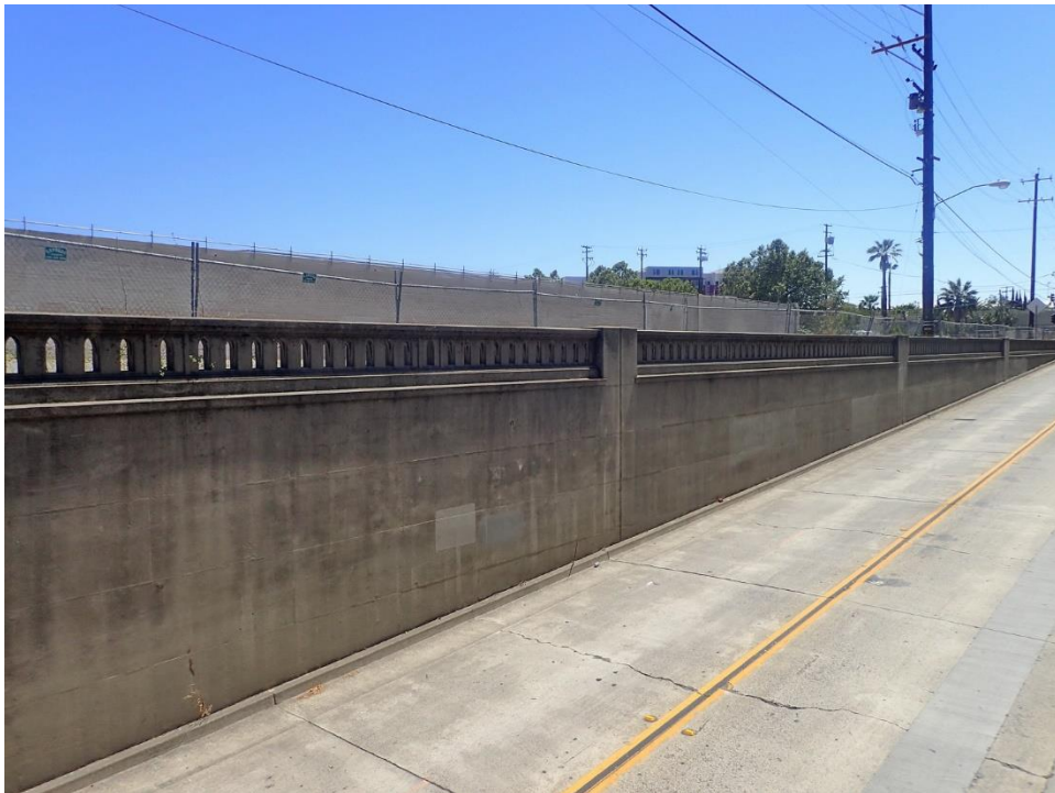
Retaining wall on southside of roadway adjacent project site.
