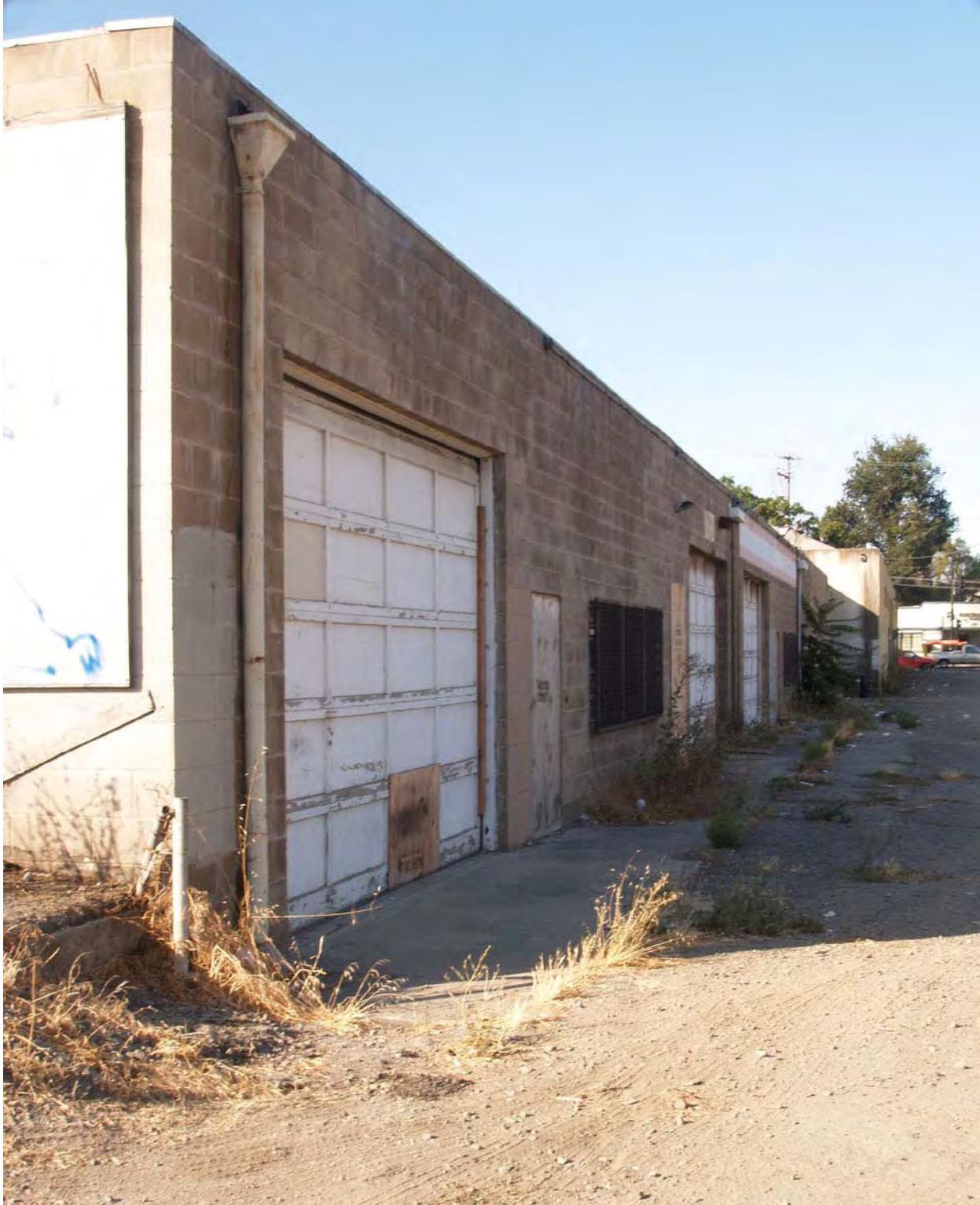
Rear building façade along West Julian Street, viewed facing southwest
