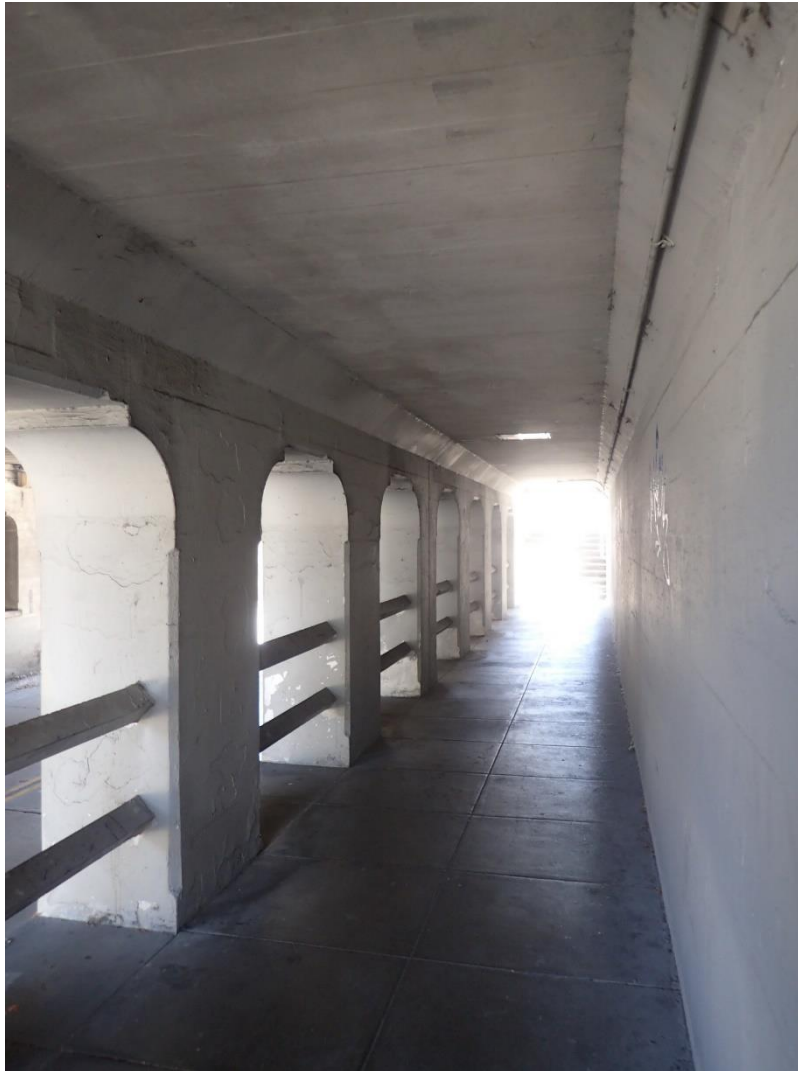
Walkway under bridge, viewed facing southwest.
