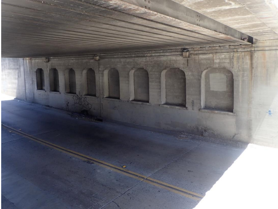
Underside of bridge on southside of roadway, viewed facing southeast
