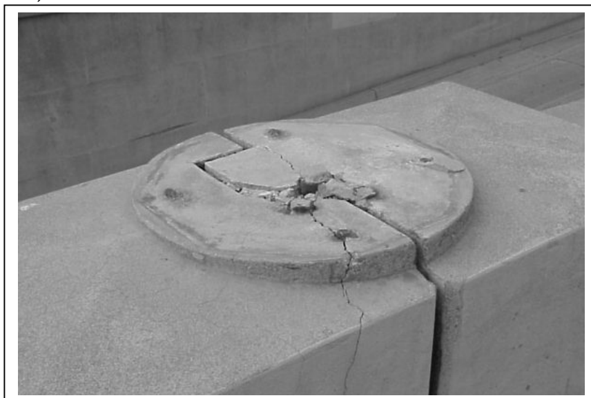
Photograph 3: Julian Street underpass, view of posts where lamps used to rest, 9/12/00
