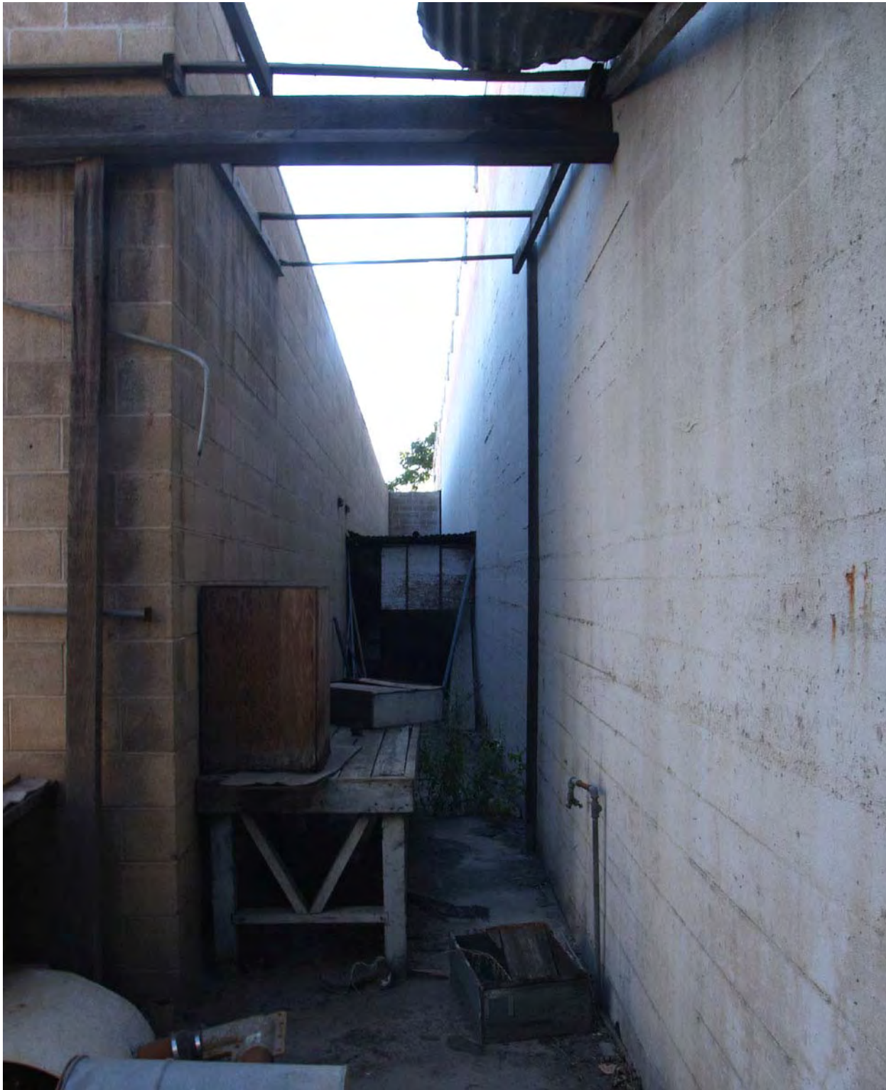
Interior space at property line, viewed facing northeast
