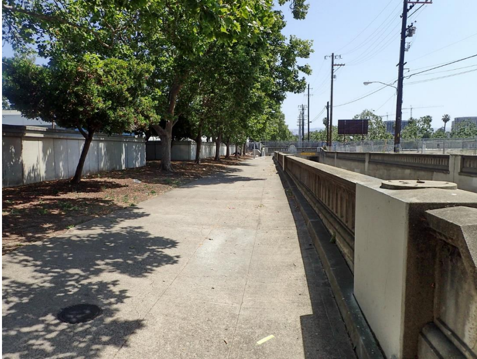
Sidewalk and railing along north side of underpass, viewed facing northeast.
