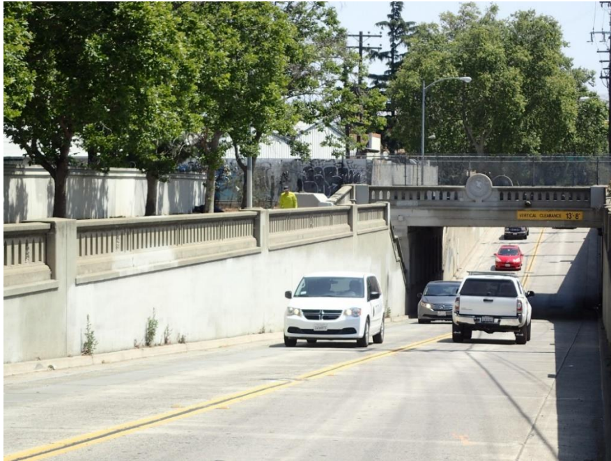
Bridge and underpass from the west entry, viewed facing northeast.
