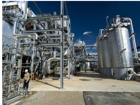
Hydrogen (green gas)
