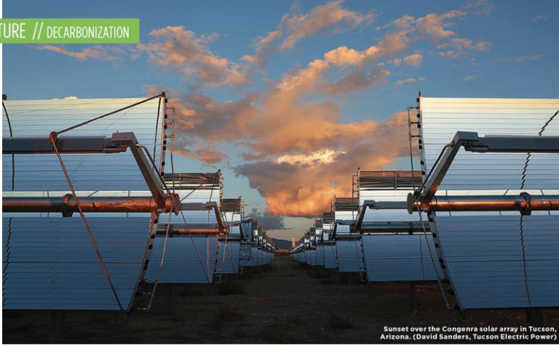
Sunset over the Congena solar array in Tucson, Arizona. (David Sanders, Tucson Electric Power)
