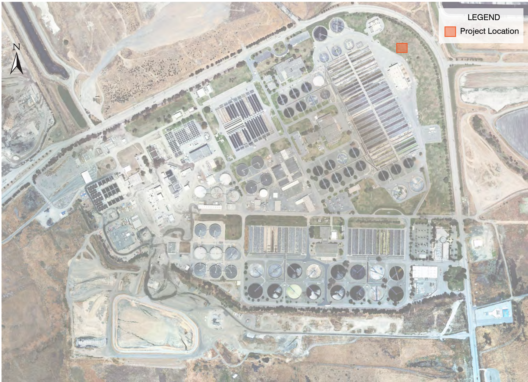
Figure 77 DIGESTER GAS STORAGE FACILITY SAN JOSÉ/SANTA CLARA WPCP MASTER PLAN CITY OF SAN JOSÉ
