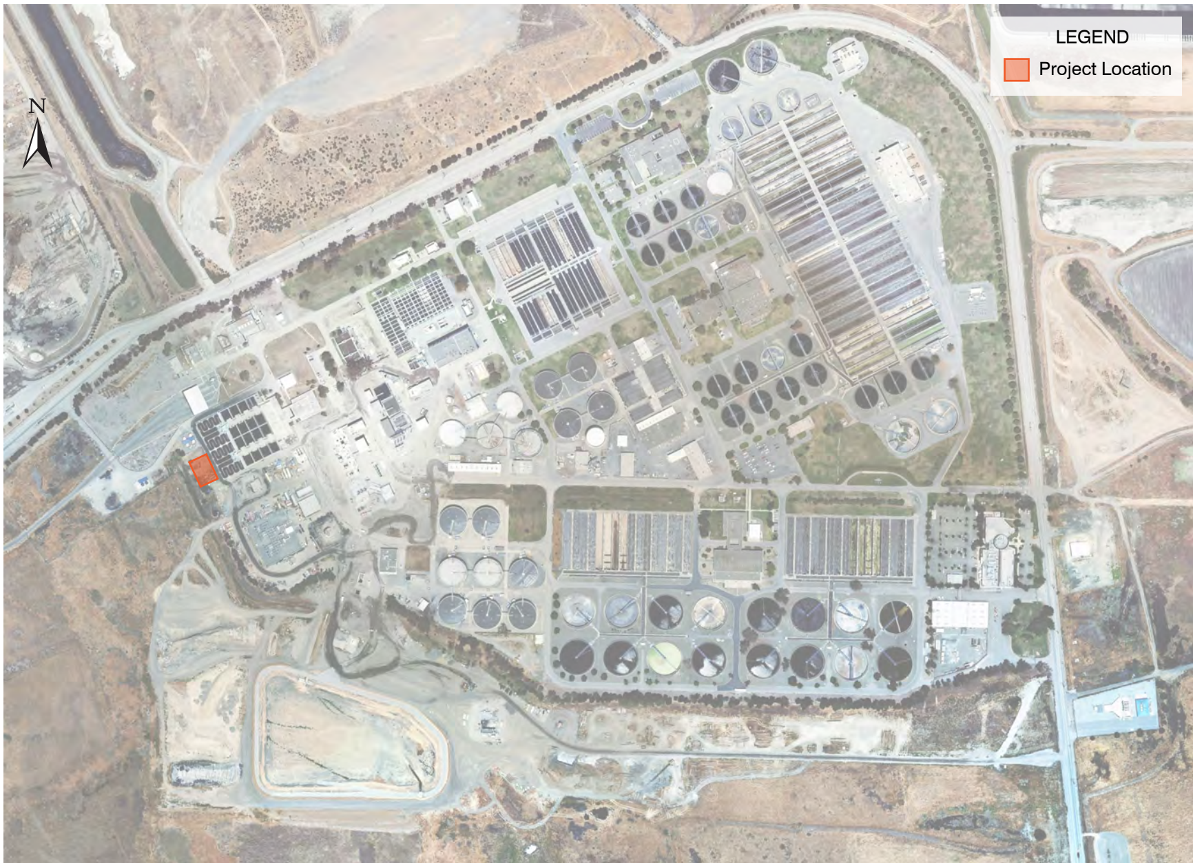
Figure 37 ADDITIONAL CHLORINE CONTACT BASINS SAN JOSÉ/SANTA CLARA WPCP MASTER PLAN CITY OF SAN JOSÉ
