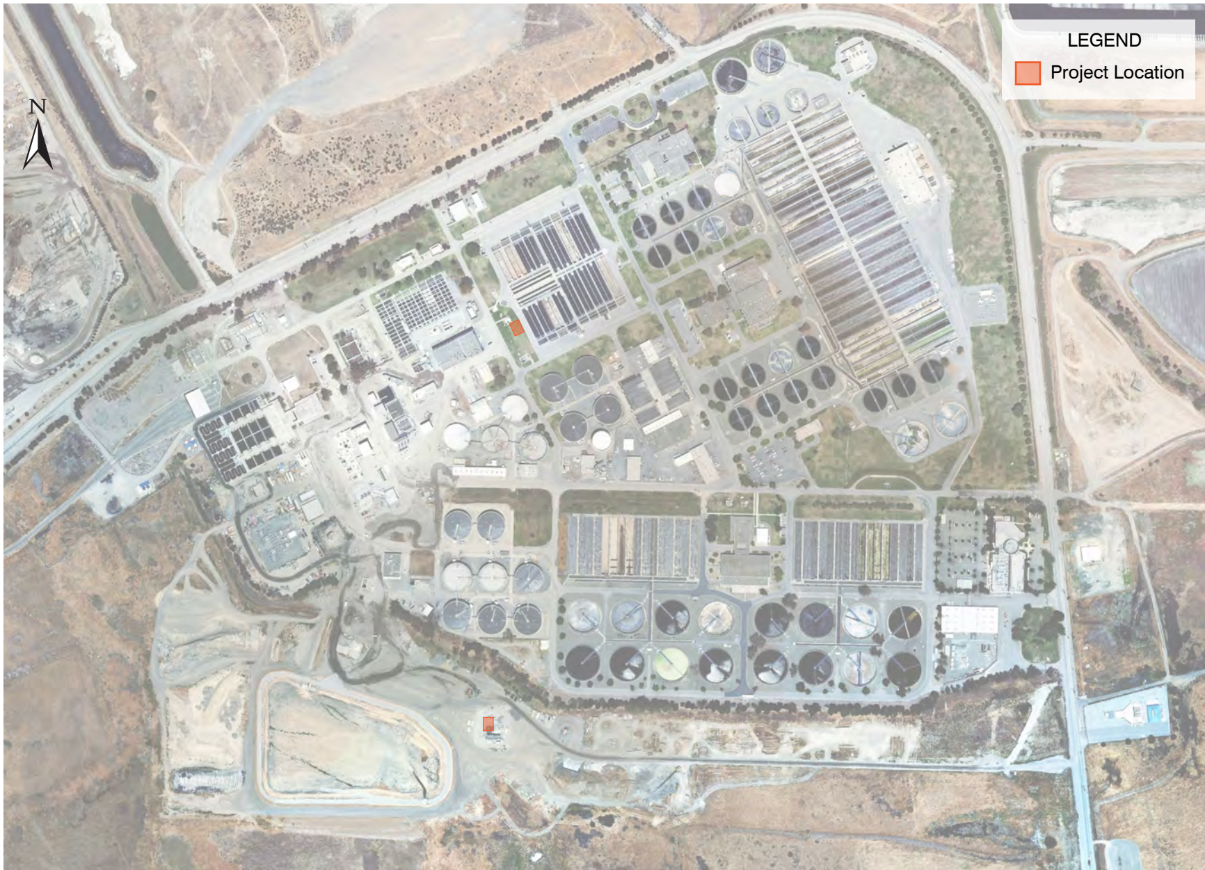
Figure 14 IRON SALT FACILITIES SAN JOSÉ/SANTA CLARA WPCP MASTER PLAN CITY OF SAN JOSÉ
