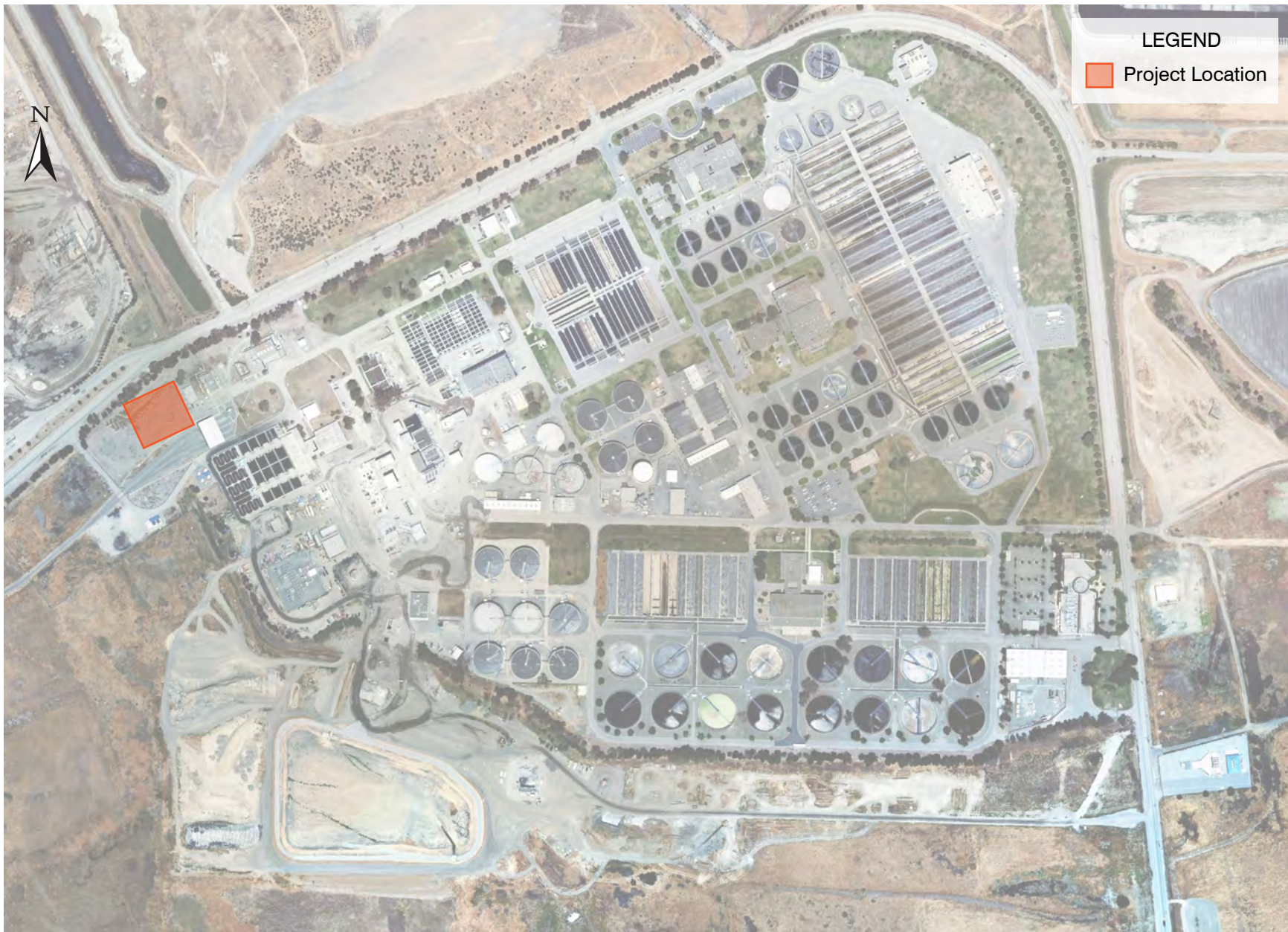
Figure 36 NEW TERTIARY FILTERS SAN JOSÉ/SANTA CLARA WPCP MASTER PLAN CITY OF SAN JOSÉ
