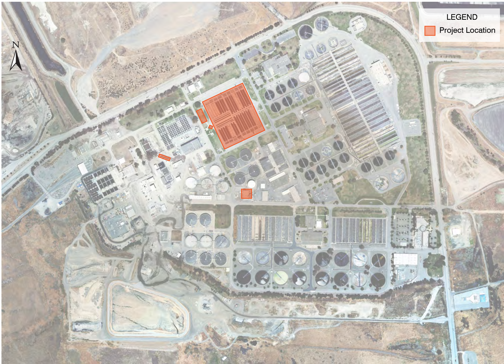
Figure 11 PRIMARY TREATMENT ODOR CONTROL SAN JOSÉ/SANTA CLARA WPCP MASTER PLAN CITY OF SAN JOSÉ
