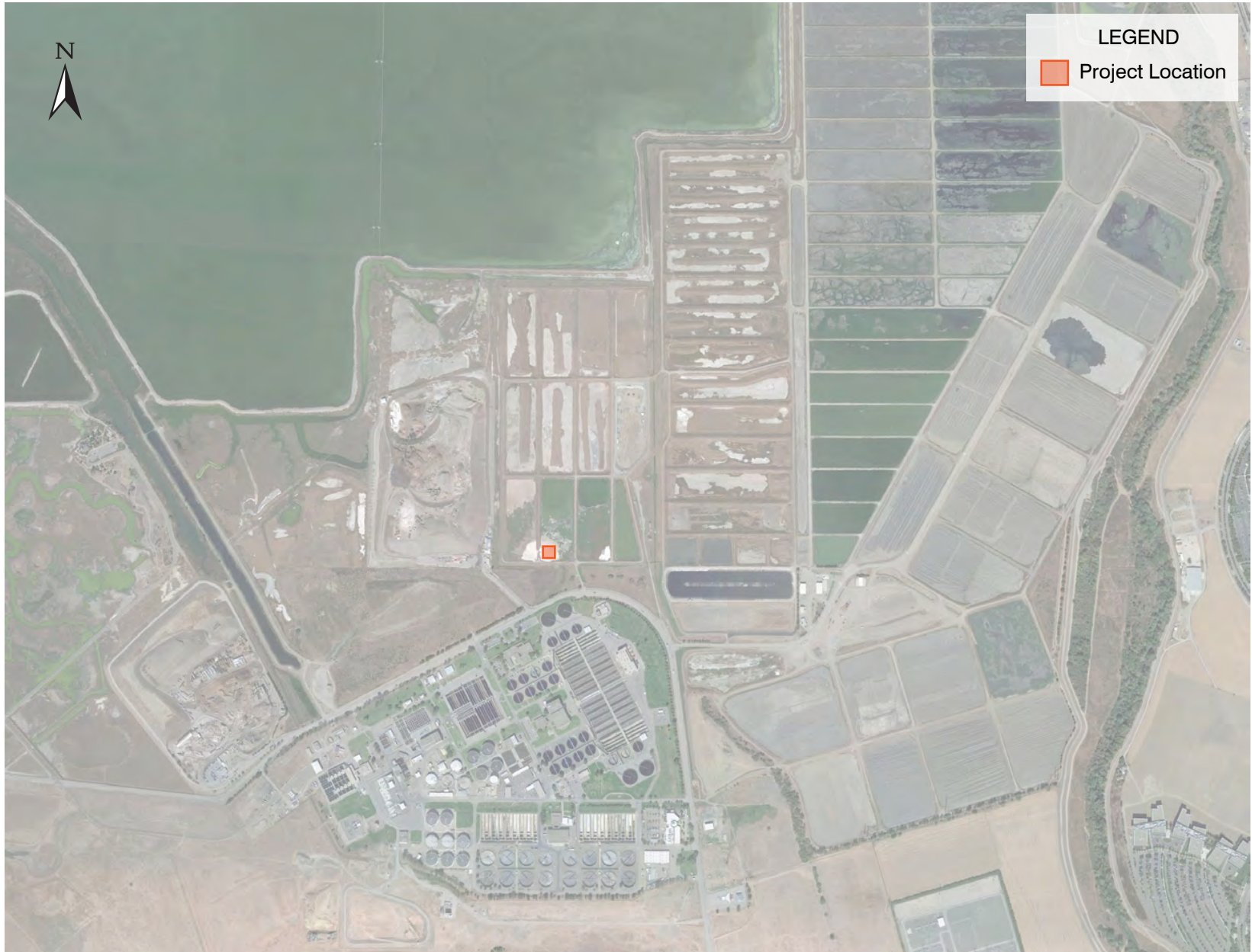
Figure 66 SLUDGE DRYING FIELD VERIFICATION SAN JOSÉ/SANTA CLARA WPCP MASTER PLAN CITY OF SAN JOSÉ
