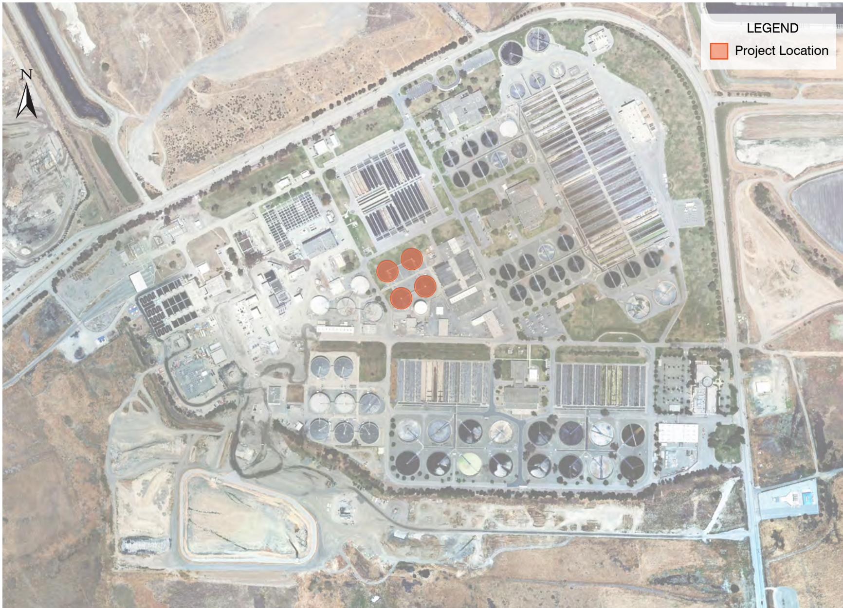
Figure 47 DIGESTER COVER AND MIXING UPGRADES (4 DIGESTERS) SAN JOSÉ/SANTA CLARA WPCP MASTER PLAN CITY OF SAN JOSÉ
