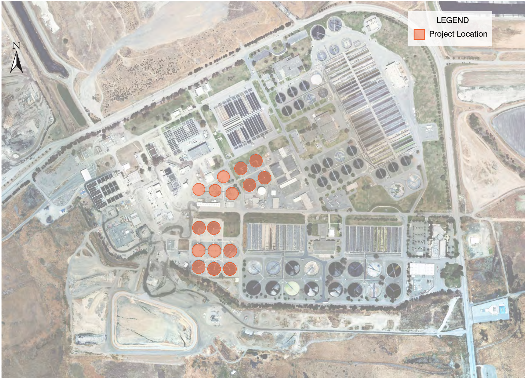
Figures 48 and 49 DIGESTER MIXING EQUIPMENT (LM MIXER AND DRAFT TUBE MIXER) SAN JOSÉ/SANTA CLARA WPCP MASTER PLAN CITY OF SAN JOSÉ
