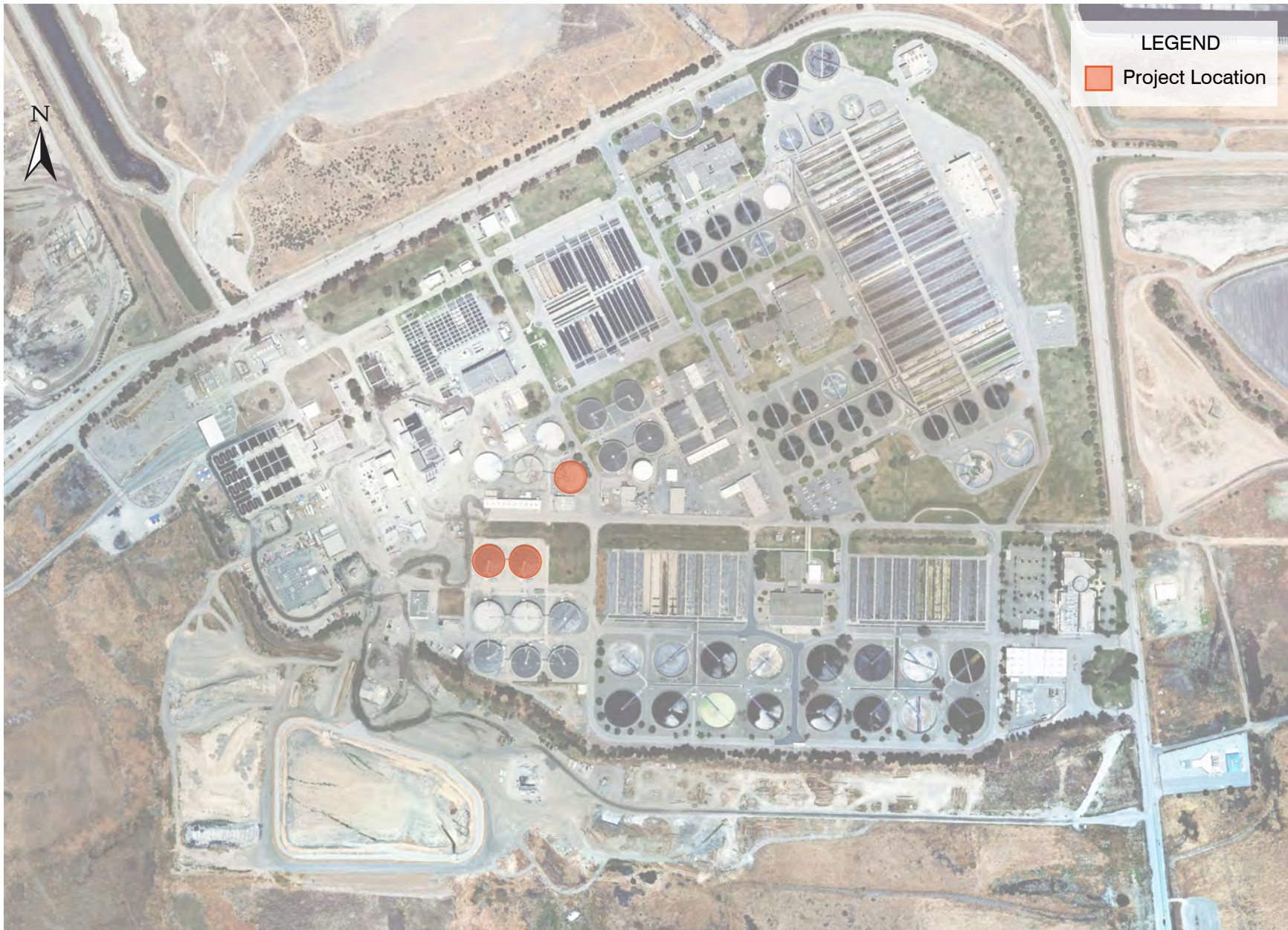
Figure 50 DIGESTER COVER AND MIXING UPGRADES (3 DIGESTERS) SAN JOSÉ/SANTA CLARA WPCP MASTER PLAN CITY OF SAN JOSÉ
