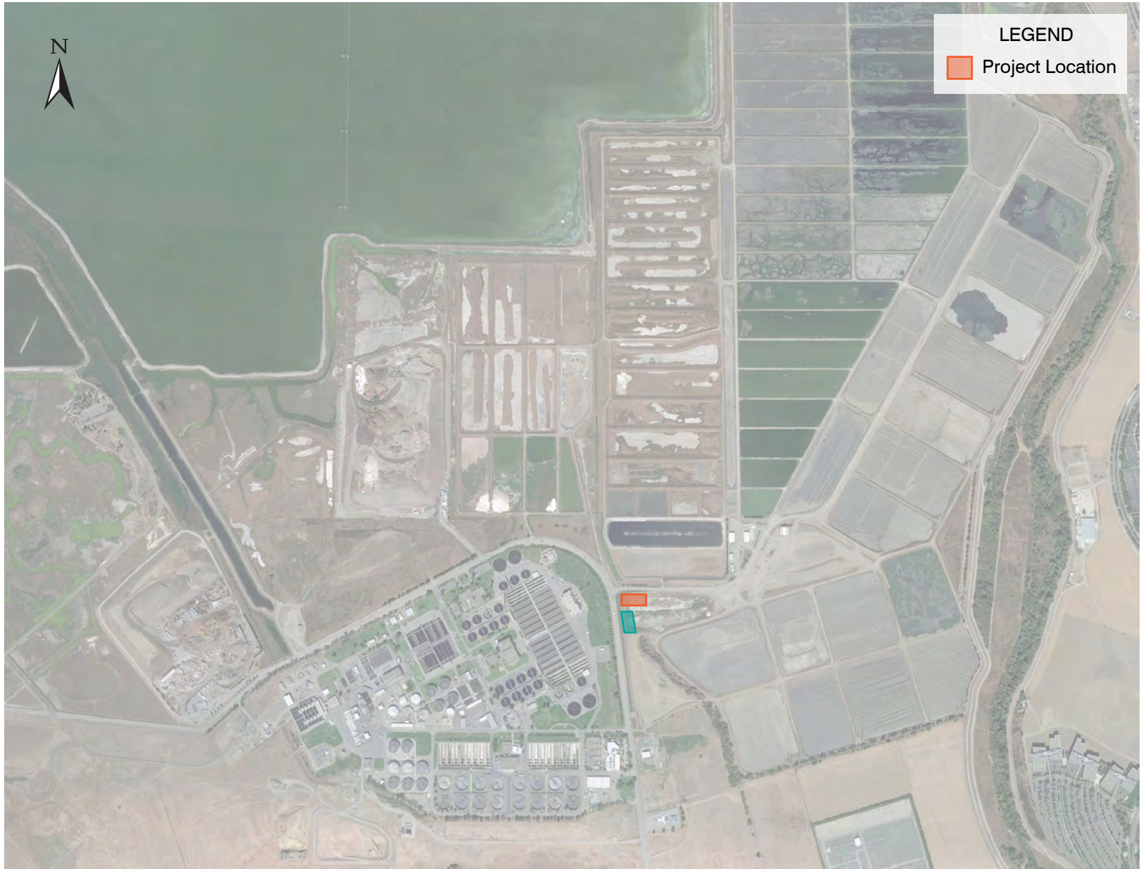
Figure 58 SLUDGE DEWATERING FIELD VERIFICATION SAN JOSÉ/SANTA CLARA WPCP MASTER PLAN CITY OF SAN JOSÉ
