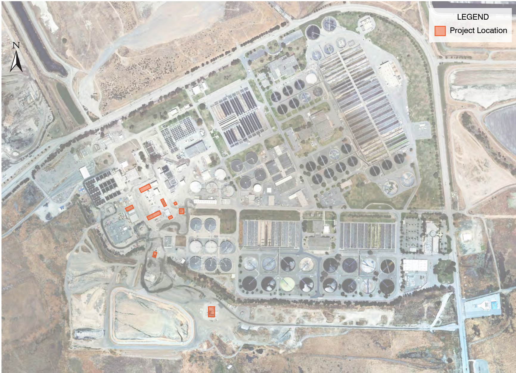
Figure 4 HEADWORKS ODOR CONTROL SAN JOSÉ/SANTA CLARA WPCP MASTER PLAN CITY OF SAN JOSÉ
