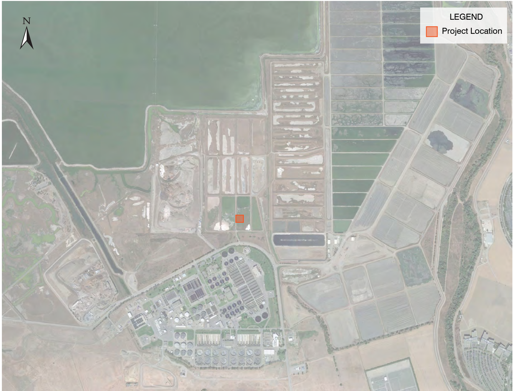
Figure 60 CAKE STORAGE SAN JOSÉ/SANTA CLARA WPCP MASTER PLAN CITY OF SAN JOSÉ
