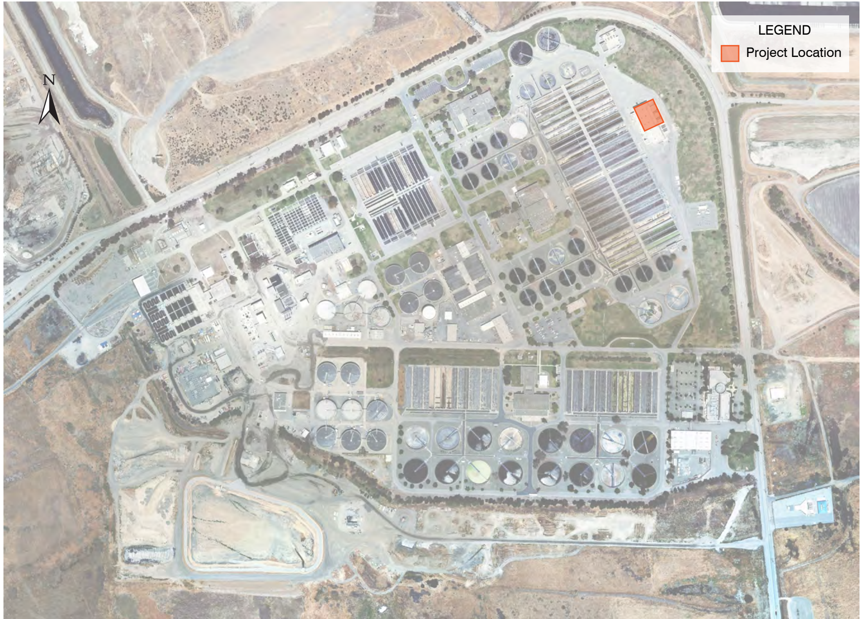
Figure 74 PLANT ELECTRICAL RELIABILITY - 4.6 MW GAS TURBINE SAN JOSÉ/SANTA CLARA WPCP MASTER PLAN CITY OF SAN JOSÉ
