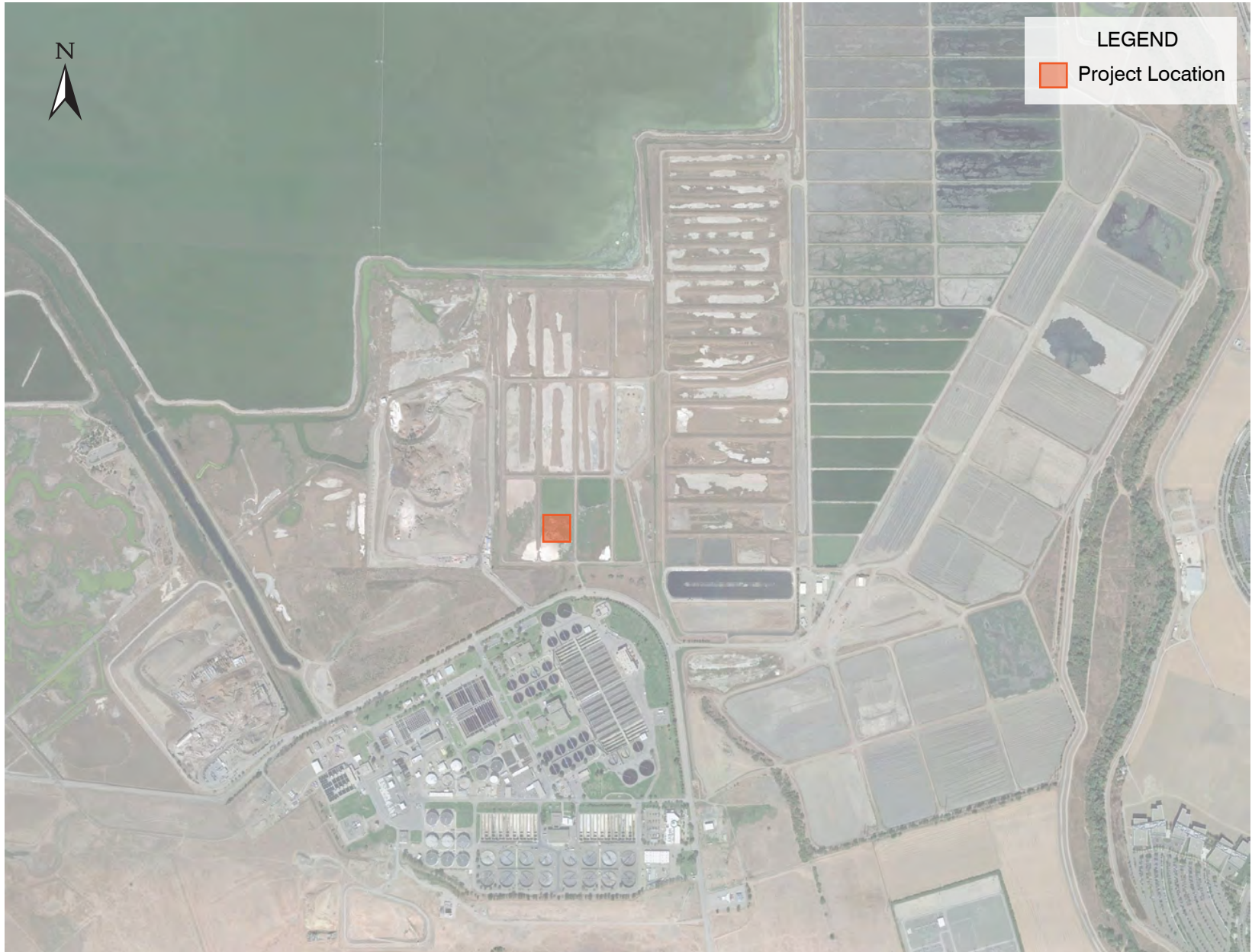
Figure 67 2/3 THERMAL DRYING SAN JOSÉ/SANTA CLARA WPCP MASTER PLAN CITY OF SAN JOSÉ
