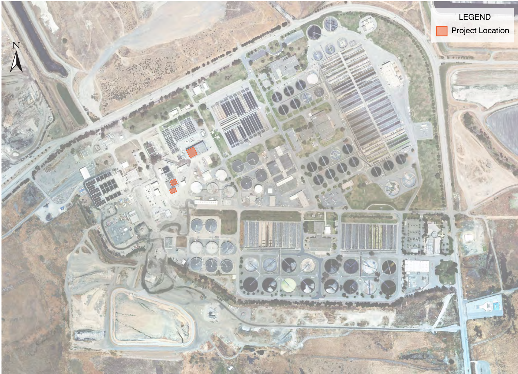
Figure 2 MISCELLANEOUS HW1 REPAIRS SAN JOSÉ/SANTA CLARA WPCP MASTER PLAN CITY OF SAN JOSÉ
