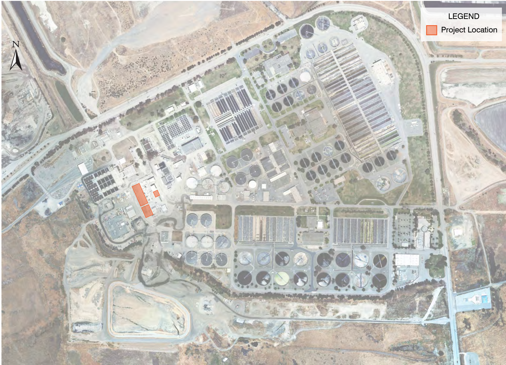
Figure 3 HEADWORKS NO. 2 MODIFICATIONS SAN JOSÉ/SANTA CLARA WPCP MASTER PLAN CITY OF SAN JOSÉ
