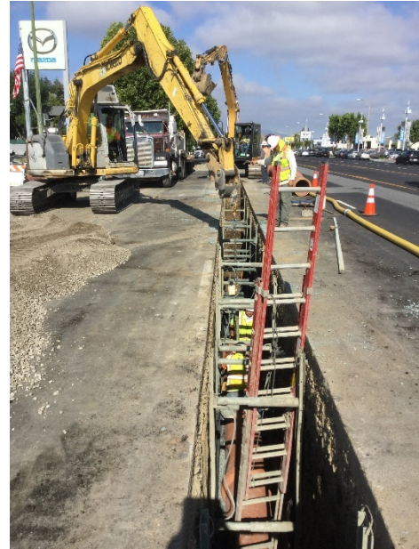
Stevens Creek Sanitary Sewer Replacement
