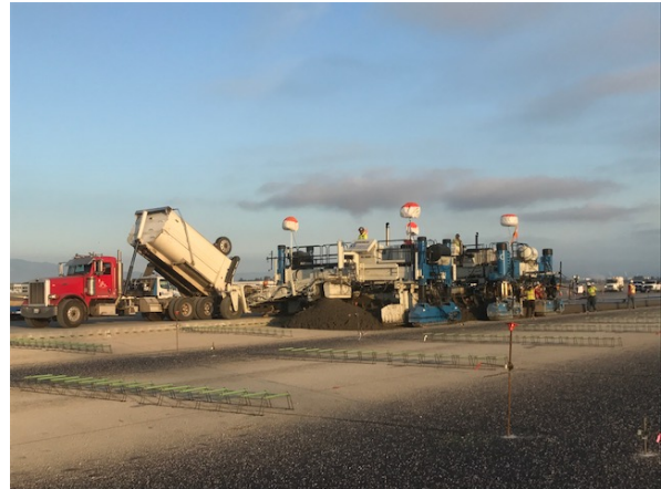
Southeast Ramp Reconstruction
