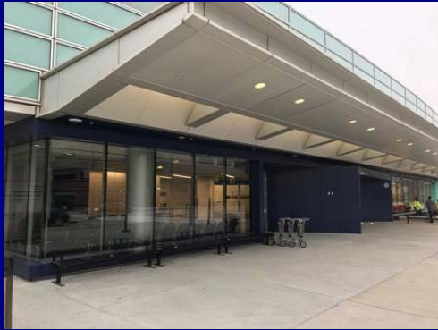
FIS Curbside Improvements
