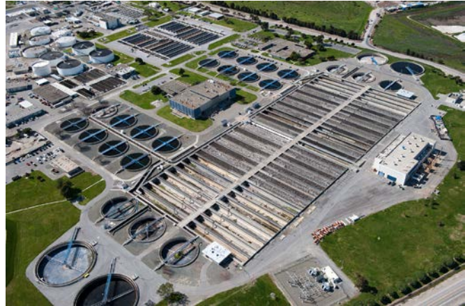
San José-Santa Clara Regional Wastewater Facility
