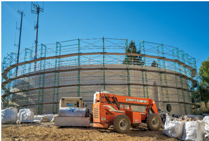
Cadwallader Tank Exterior
