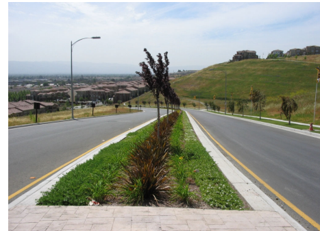
Median Island at Communication Hill
