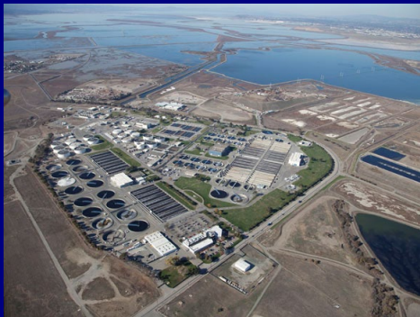
Water Pollution Control Plant
