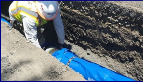
New Water Main Pipe Installation at Gumdrop Drive
