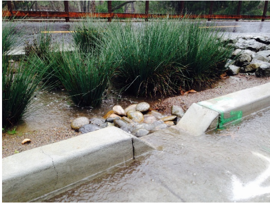
Example of a Stormwater Bioretention Treatment Facility in South San José
