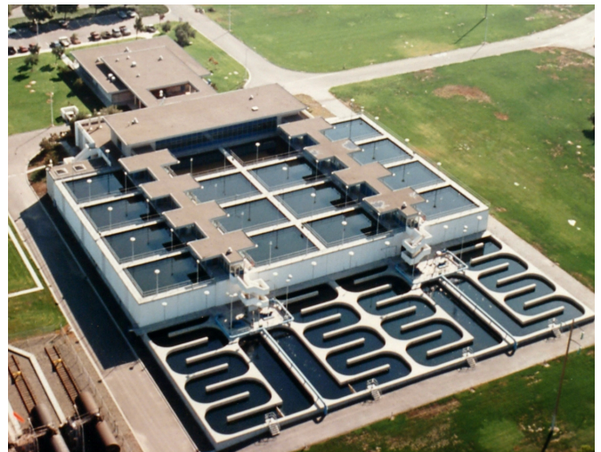
Aerial of Filter Building
