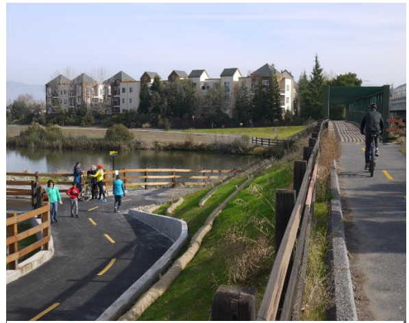
Coleman Road Under-crossing
