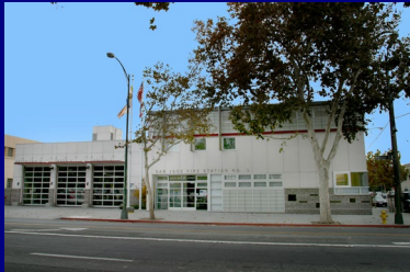
Major Repairs at Fire Stations 3, 4, 9 and 30
