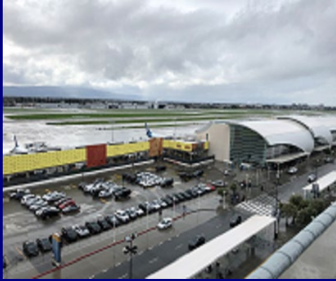
Interim Terminal Facility
