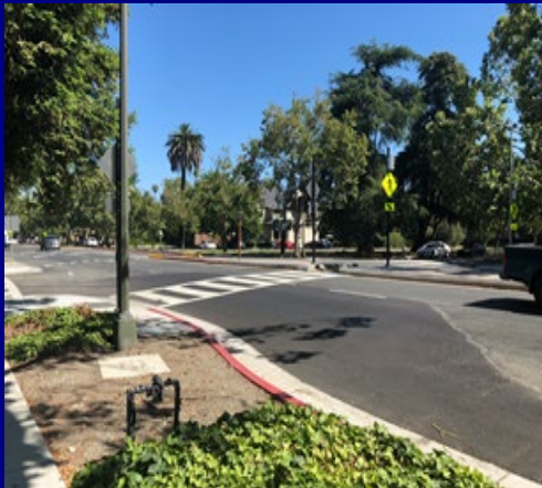
Pedestrian Safety Improvements at the Alameda and Emory St.
