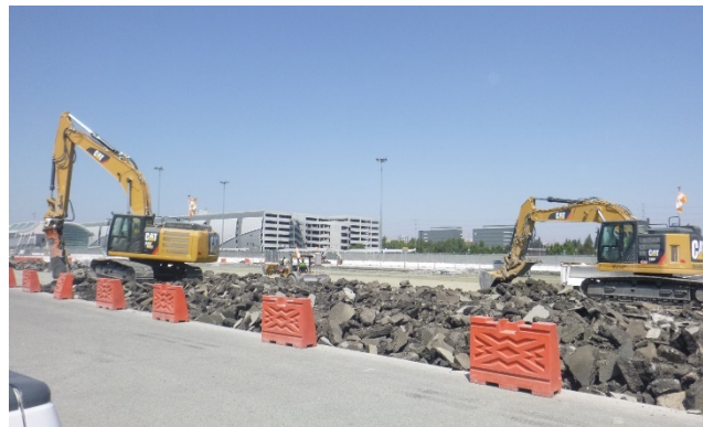
Terminal B Ramp Rehabilitation
