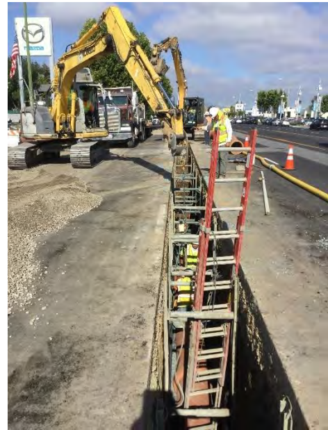
Stevens Creek Sanitary Sewer Replacement
