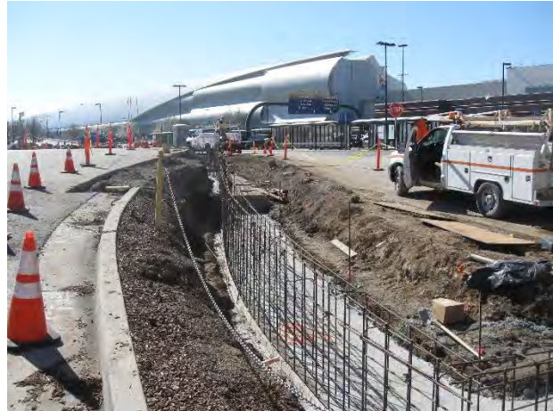
Terminal A Ground Transportation Island
