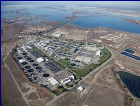
Water Pollution Control Plant
