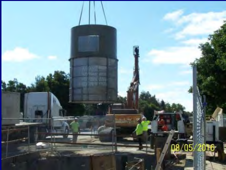
Large Trash Capture Device Installation
