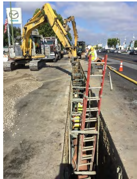
Stevens Creek Sanitary Sewer Improvement
