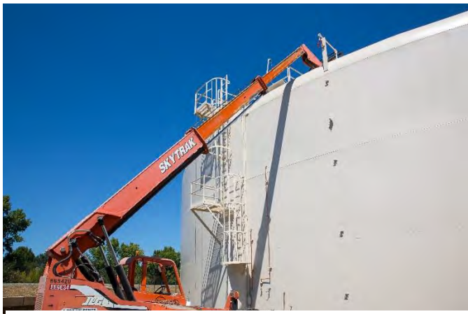
Detail Work on Trimble Reservoir
