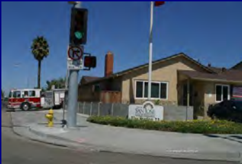
Major Repairs at Fire Stations 18 and 23
