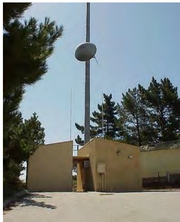
Cadwallader Reservoir Radio Tower
