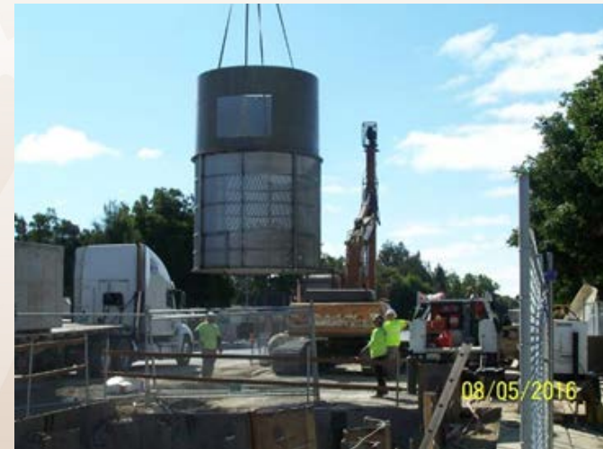
Large Trash Capture Device Installation
