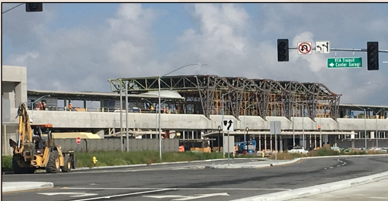
BART Berryessa Station Construction
