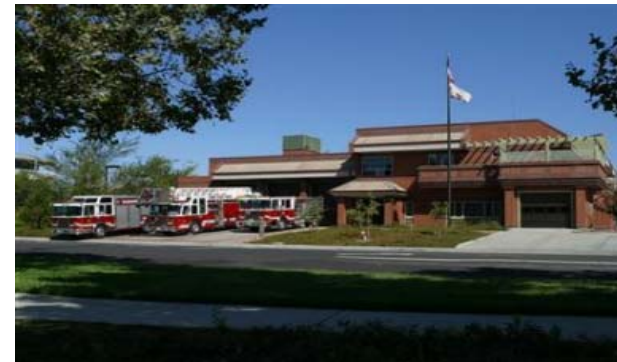
Fire Station 29 Generator Replacement
