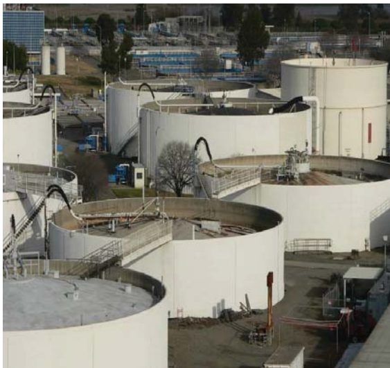
Existing Digester Facilities
