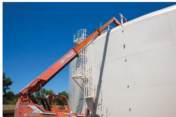
Detail Work on Trimble Reservoir
