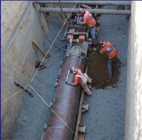
Almaden Expressway Sanitary Sewer Improvement Project (Bore and Jack Operation)
