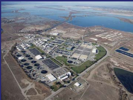
Water Pollution Control Plant
