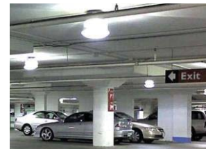
LED Garage Lighting Upgrades
