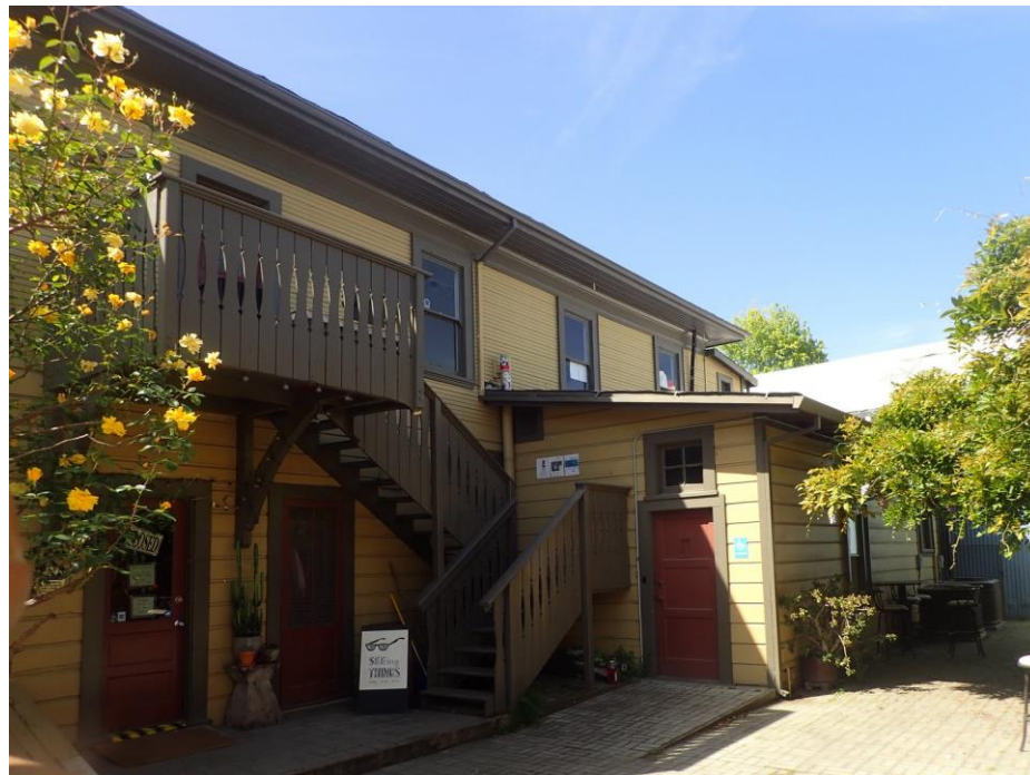
Rear elevation of Locurto Store building, viewed facing southwest.
