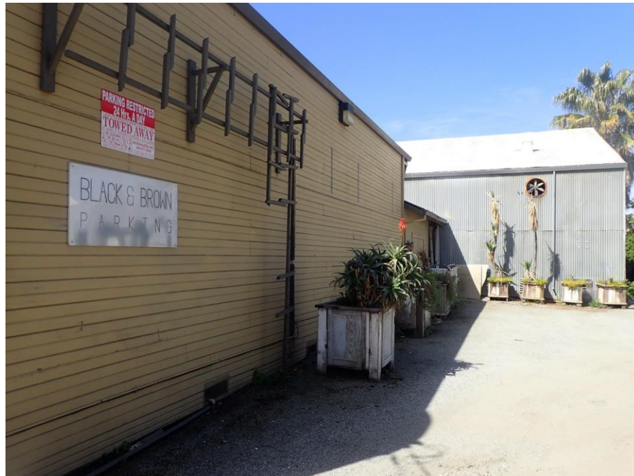
North elevation of clubhouse, viewed facing west.
