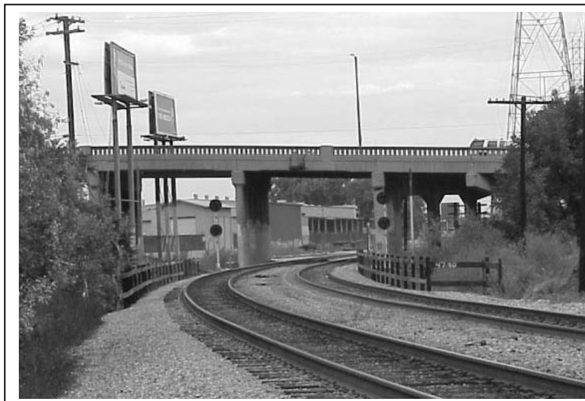
Photograph 2: Carlos Street Overpass, camera facing north, 9/12/00.
