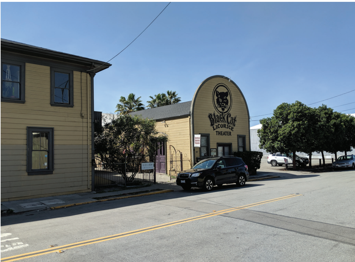
Photo 4.1-6 – Gallery, theater, and retail uses west of project site.
