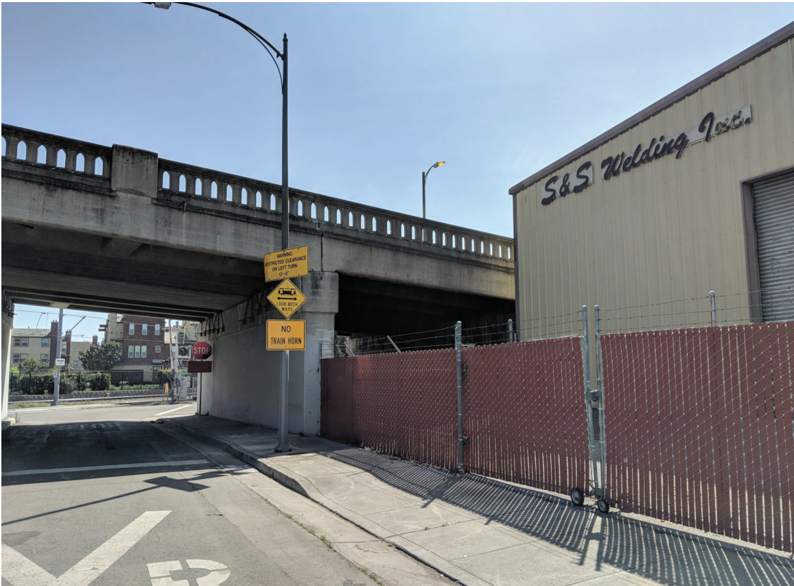
Photo 4.1-5 – West San Carlos Street bridge ramp south of project site.
