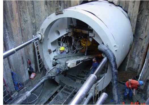
Rincon Storm System Improvements, Phase II
