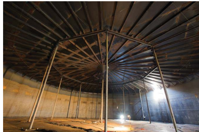
Interior of Cadwallader Reservoir
