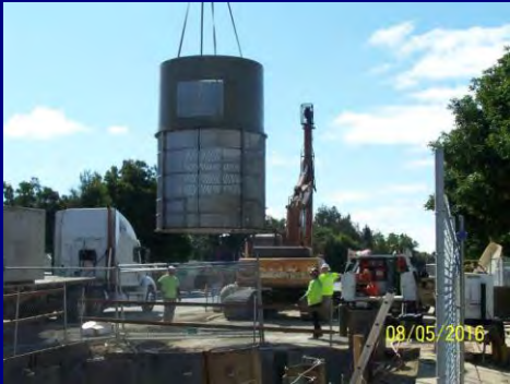
Large Trash Capture Device Installation
