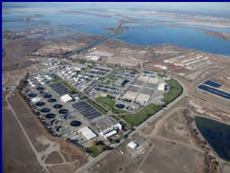
Water Pollution Control Plant
