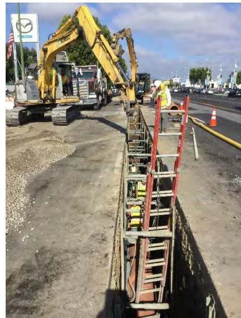
Stevens Creek Sanitary Sewer Improvement
