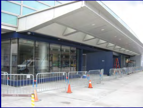
FIS Curbside Improvements
