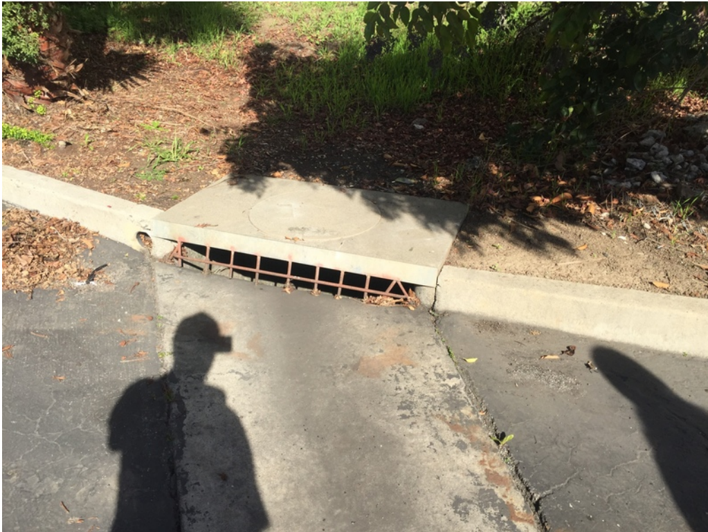
Stormdrain located on eastern corner of property
