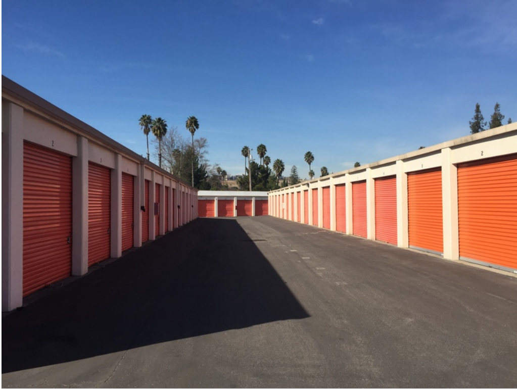
Driveway showing entrances to various storage units facing east
