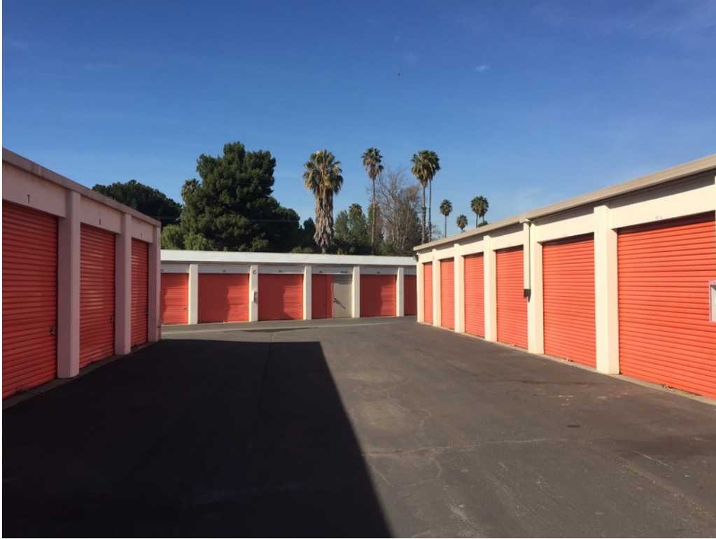
Storage units driveway facing east 16
