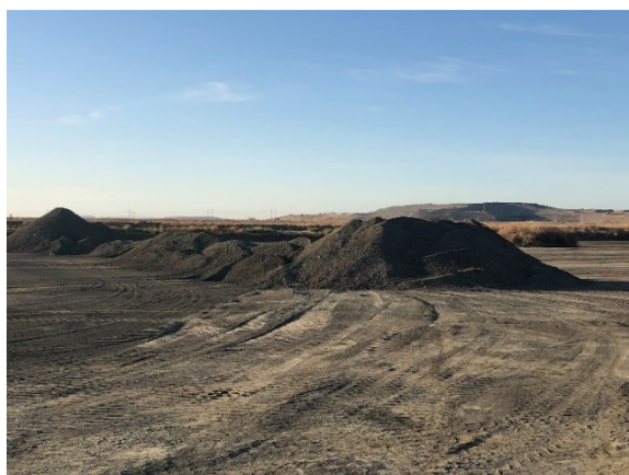
FIGURE 5 BIOSOLIDS SOLAR-DRIED, PILED, AND READY FOR HAULING FOR USE AS ALTERNATE DAILY COVER
