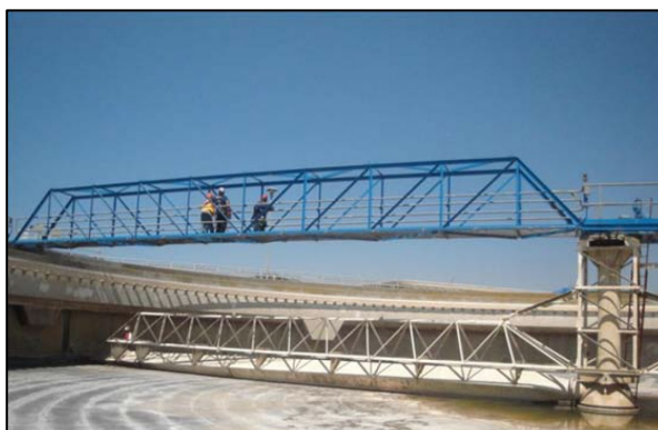
FIGURE 45 WORKER ON A CLARIFIER "TOW-BRO" ARM
