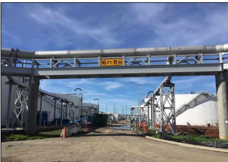
FIGURE 42 NEW PERMANENT ABOVE-GROUND PIPING RACKS: “THE MONORAIL” AT THE REMOTE DIGESTERS
