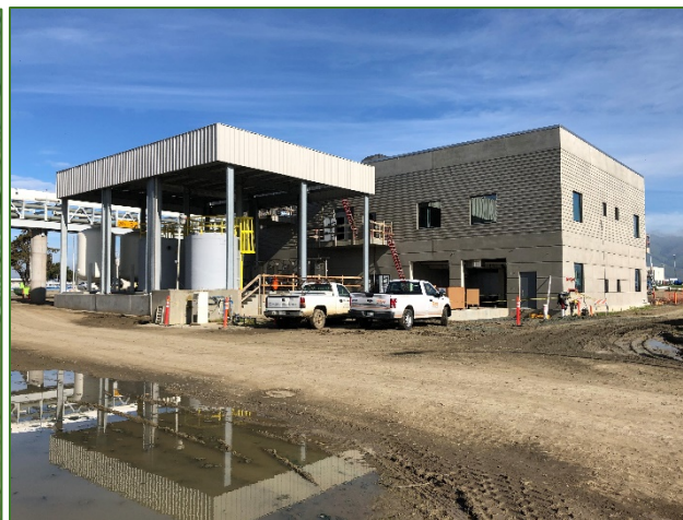
FIGURE 40 NEW SLUDGE SCREENING BUILDING NEARING COMPLETION
