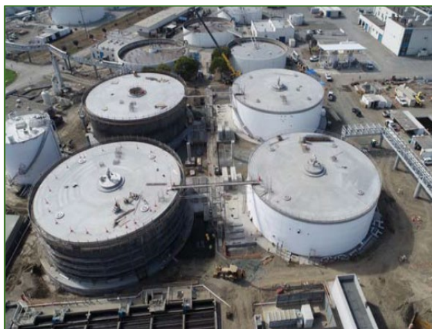
FIGURE 41 AERIAL IMAGE OF PROGRESS ON UPGRADES TO DIGESTERS 5 - 8
