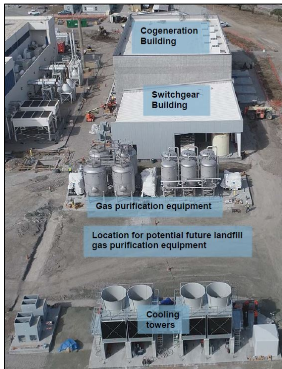
FIGURE 30 OCTOBER 2019: CONSTRUCTION OF THE NEW COGENERATION BUILDING
