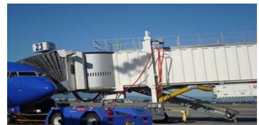
Jet Bridge Refurbishment
