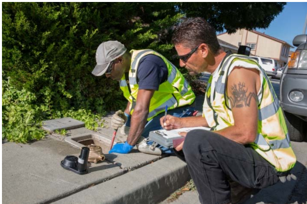
Meter Replacement Project
