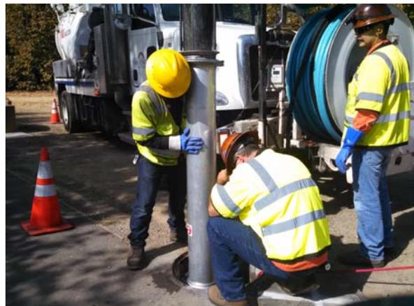
***Clean-Out of a Continuous Deflective Separation unit installed in the Selma Olinder neighborhood***
