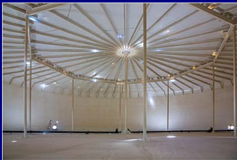
Interior of Trimble Reservoir
