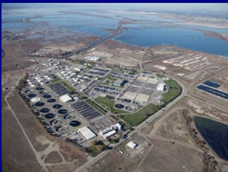
Water Pollution Control Plant
