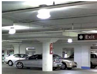
LED Garage Lighting Upgrades
