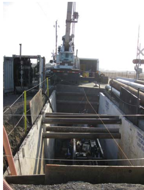
Sewer Rehabilitation by Bore and Jack Operation
